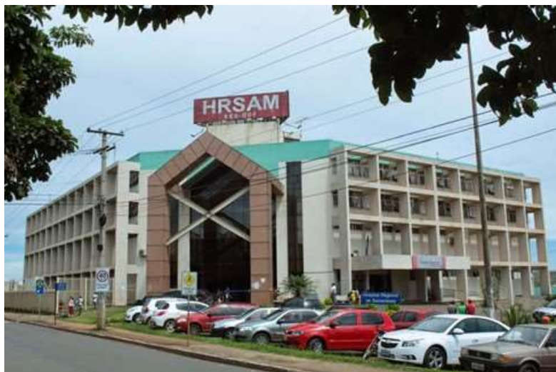
HOSPITAL REGIONAL DE SAMAMBAIA
